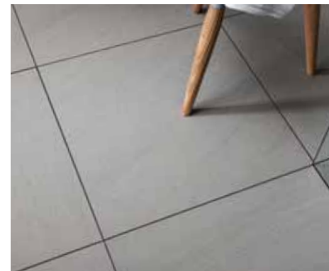
Floor tile grout
